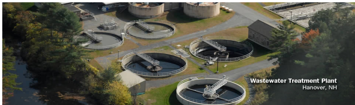
Above: Hanover Wastewater Treatment Plant
